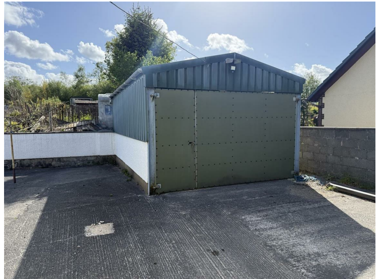
Detached Garage / Workshop
